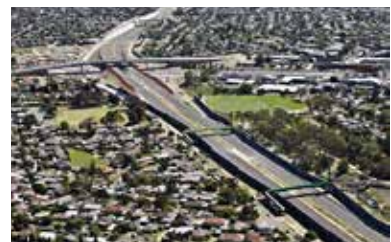
Figure 10 Freeways often create walking barriers between urban areas
